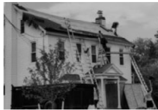
New roof being put on Parish Office by Mike Peter’s Roofing
